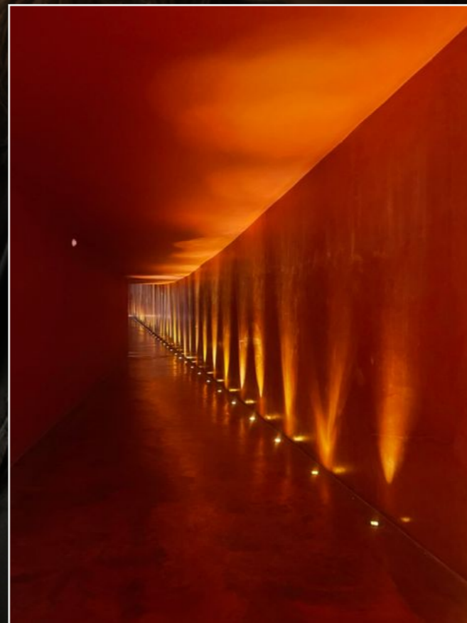
Recessed floor lighting
